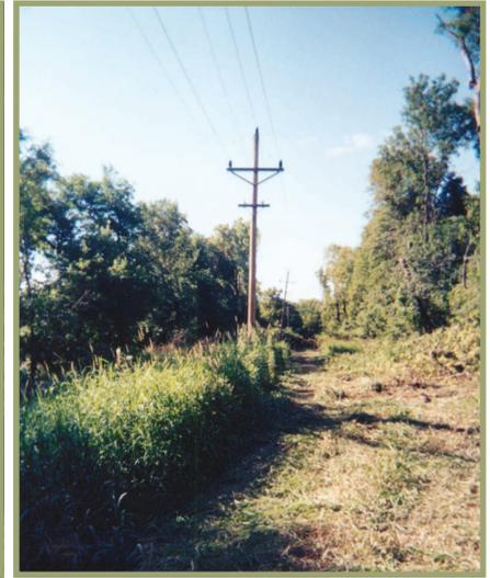
**P**roper tree clearance around power lines
