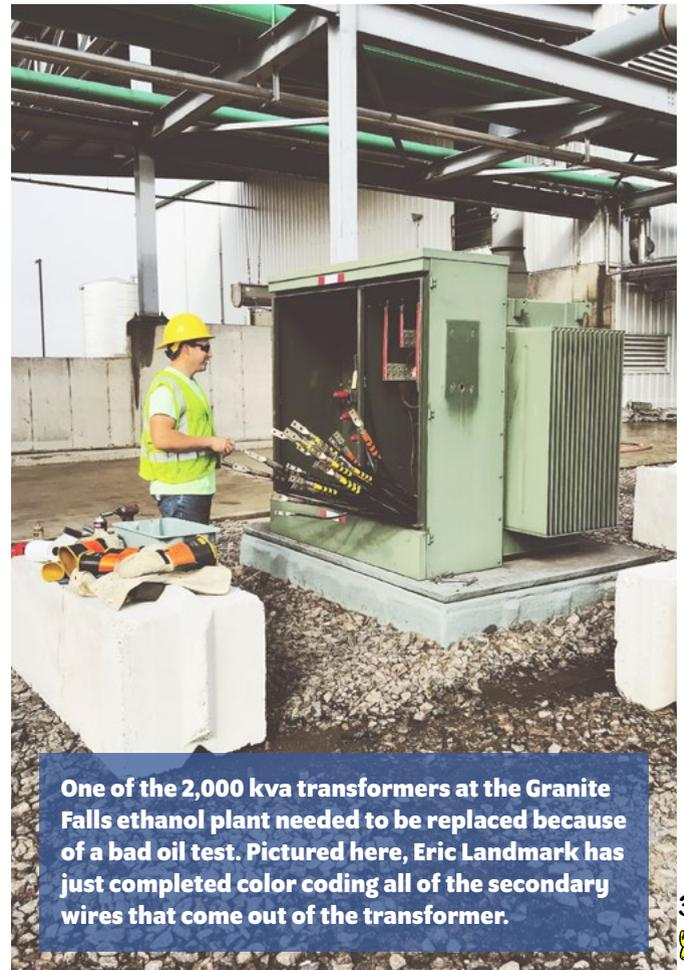
**One of the 2,000 kva transformers at the Granite Falls ethanol plant needed to be replaced because of a bad oil test. Pictured here, Eric Landmark has just completed color coding all of the secondary wires that come out of the transformer.**
