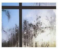
If the condensation occurs on the prime window and the window is double-glazed, that usually means the relative humidity is too high for the temperature conditions. With a thermostat set at 70 degrees, condensation should
