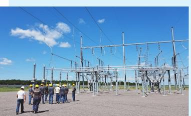
The original F.L Blair Substation had exceeded its service life and needed to be rebuilt to increase reliability and operability, as well as to accommodate the connection of new wind generation via the Otter Tail Power Company interconnection. Work on the rebuild began in March 2019 and wrapped up in July 2019.
