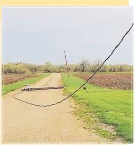
left us with no feed to the Watson, Rosewood, Gluek and Asbury Substations. Poles replaced near Asbury gave us a source to feed these substations.
